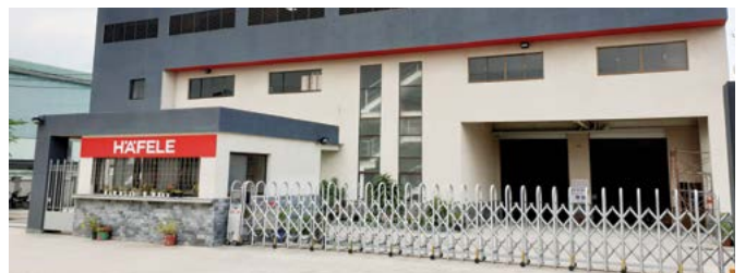
Häfele Production Plant Binh Duong, Vietnam
